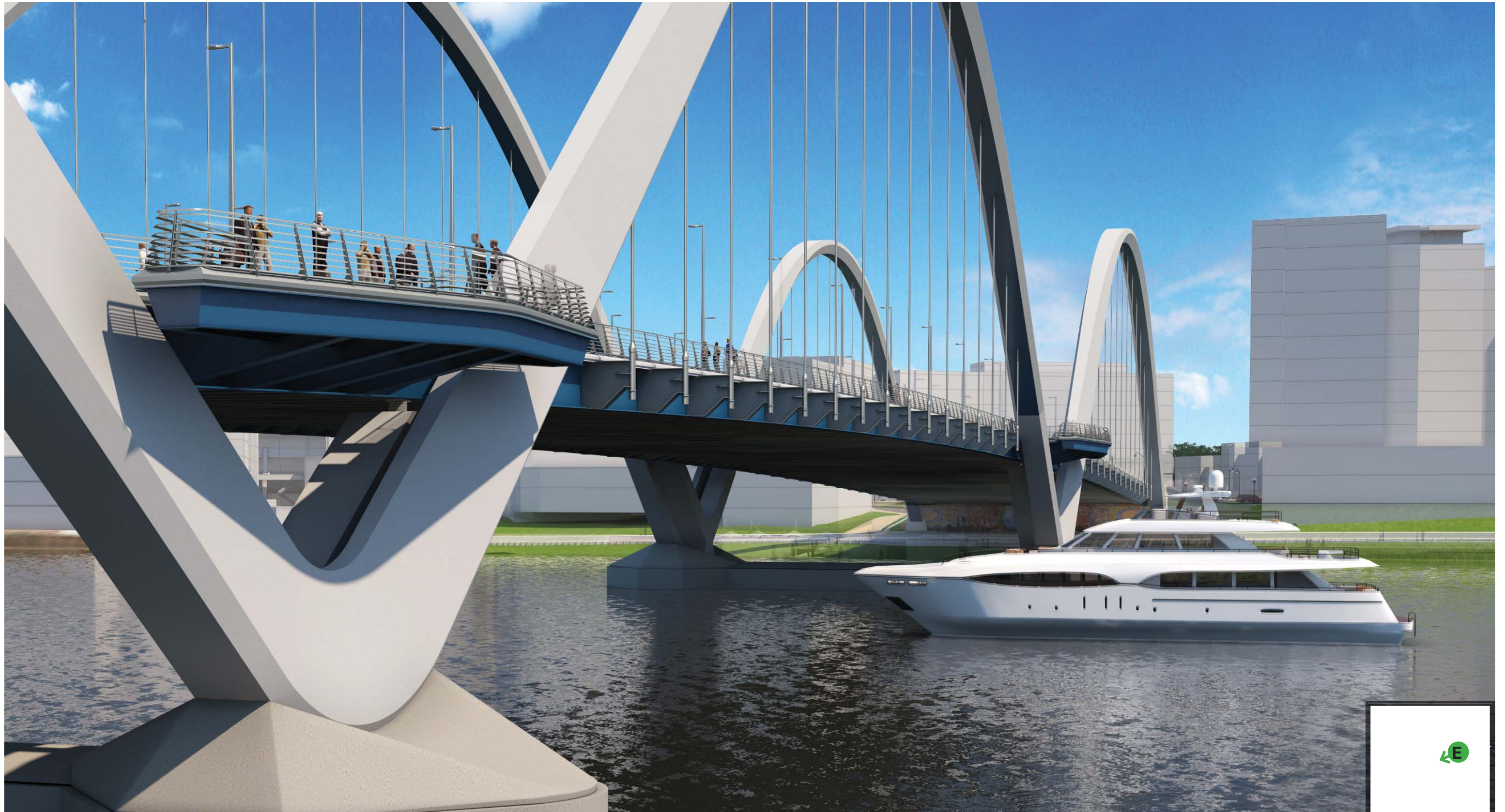
The v-piers seamlessly contribute to the geometry of the arches and result in the arches “springing” off the water.
