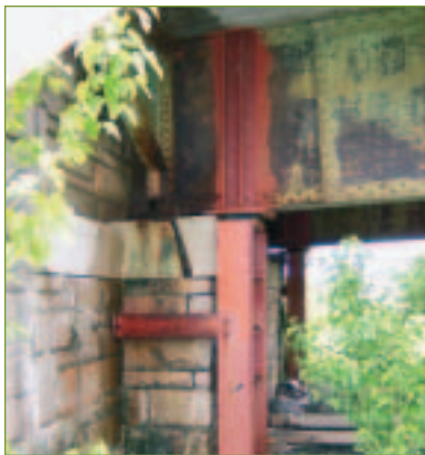
Frederick Douglass Memorial Bridge failed bearing plate at southeast abutment
