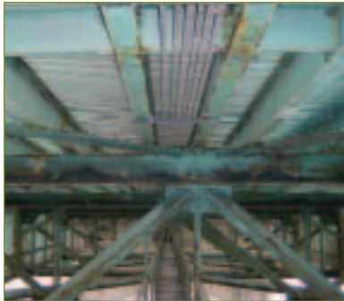
Steel corrosion in the Frederick Douglass Memorial Bridge structure
