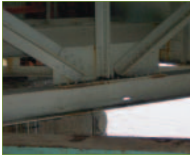
Frederick Douglass Memorial Bridge steel section loss
